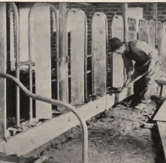
Placing the concrete manger curb.
